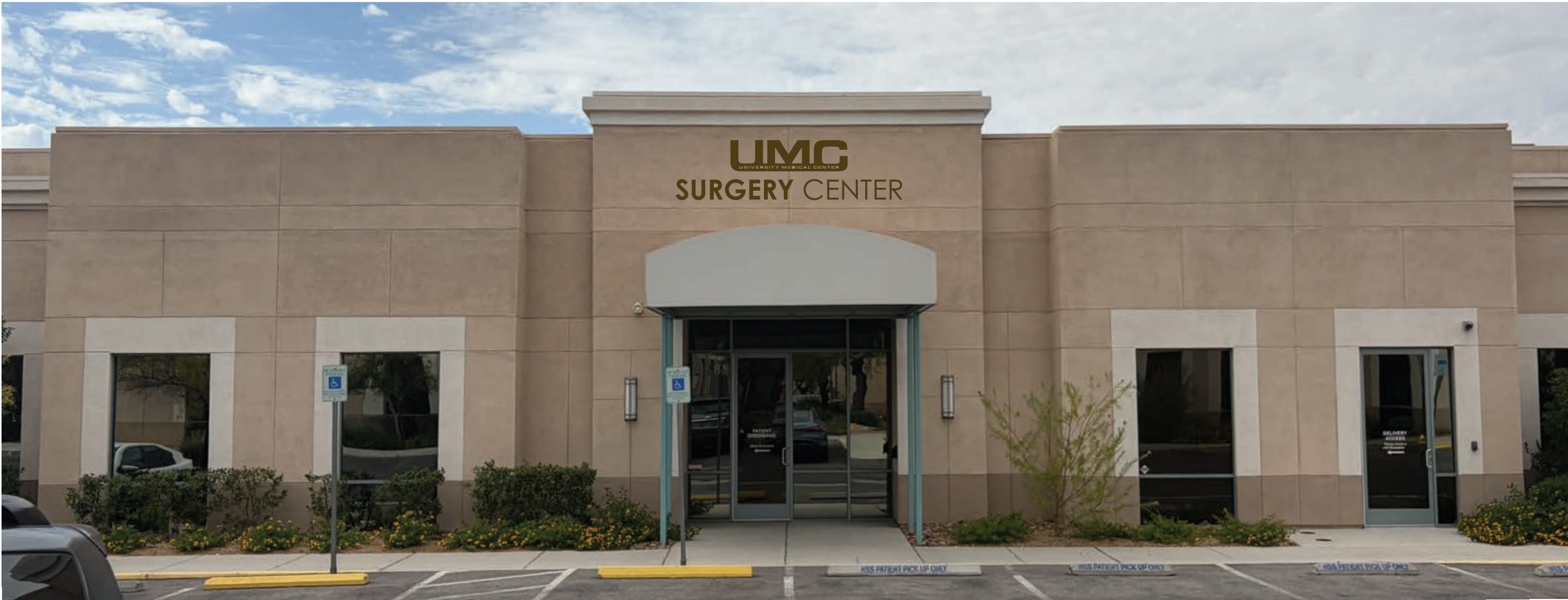
North Elevation Entrance 2
