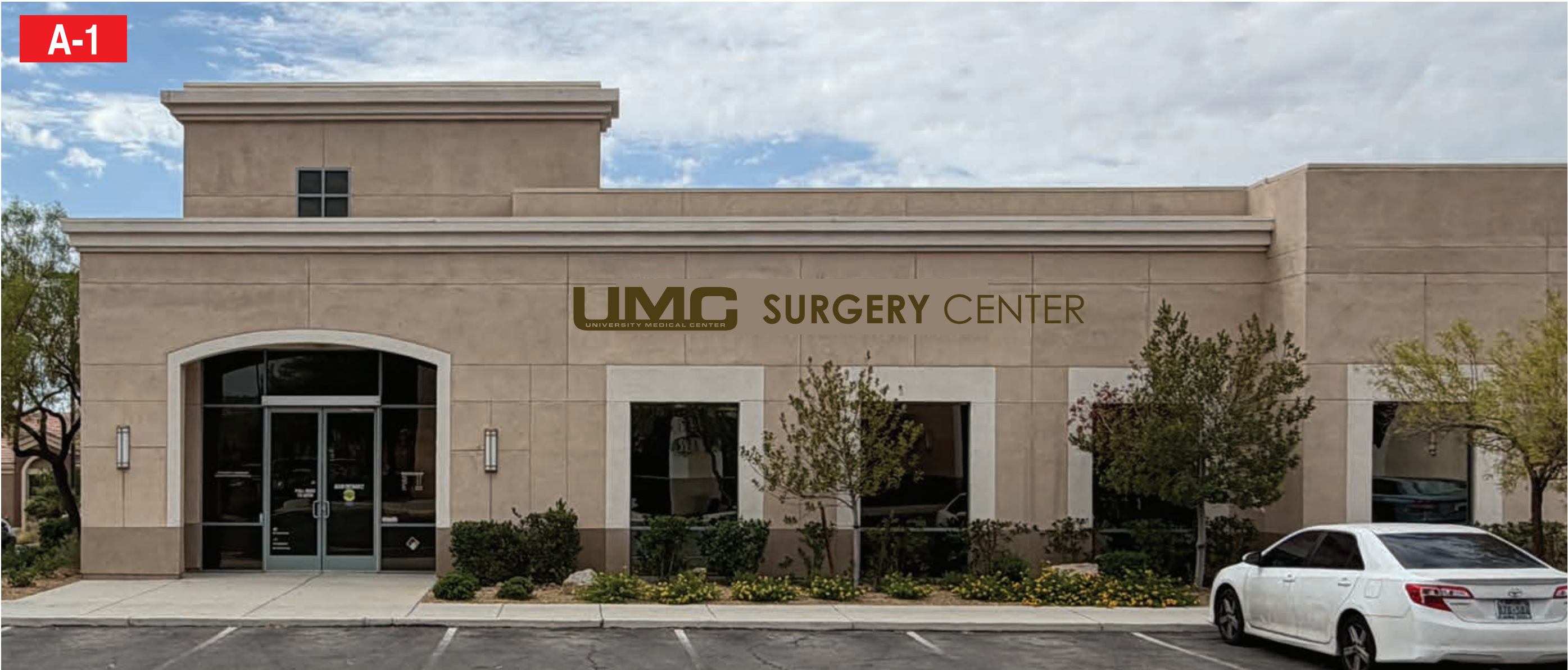
North Elevation Entrance 1
